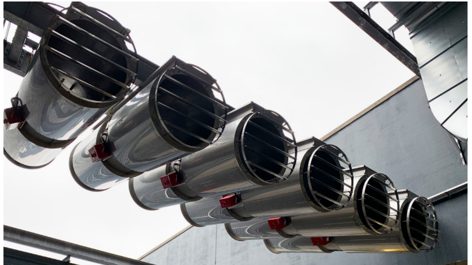
NOVENCO AUR tunnel jet fans in the Heinenoord Tunnel
