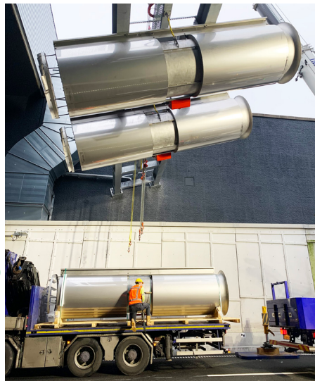
Installation of NOVENCO fans along the tunnel ceiling for ventilation and smoke control
