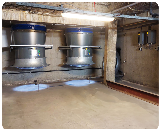
Post-installation: Compact, energy-efficient ZerAx fans
