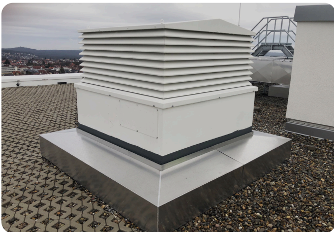
Rooftop louvre hood with high-speed actuator, designed for 0.7-second response, ensuring immediate airflow regulation and system stability
