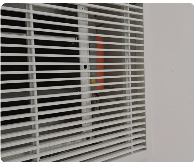
Corridor-mounted combination damper and outlet grille, delivering precise airflow and homogeneous pressure as part of the system
