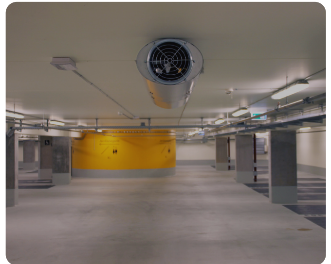
Installation with NOVENCO jet fan AUO
