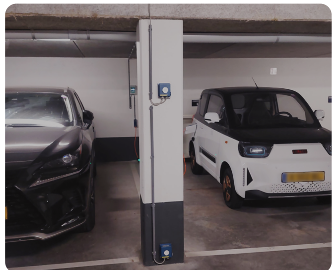
CO/LPG detection system for continuous monitoring and safety
