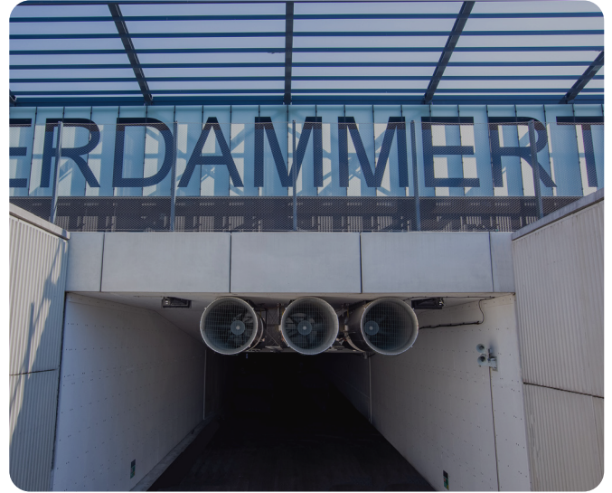
Entrance of the Gaasperdammertunnel
