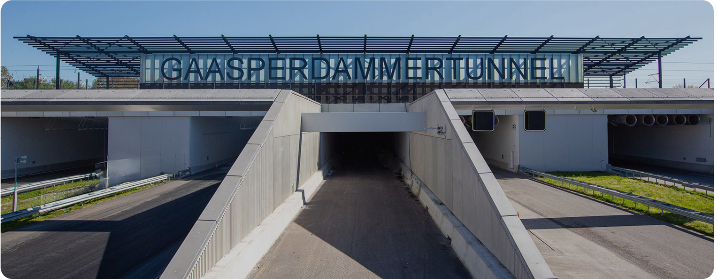
Gaasperdammertunnel, The Netherlands
