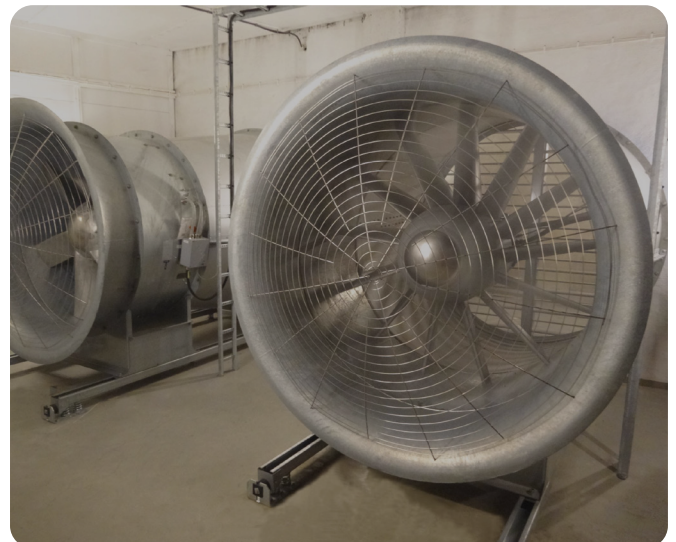
New fans installed – cutting energy use by over 30%
