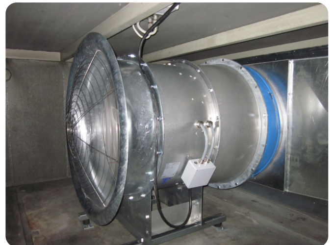
New installed ZerAx fan replacing two old units
