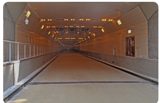
One of the Maastunnel entrances
