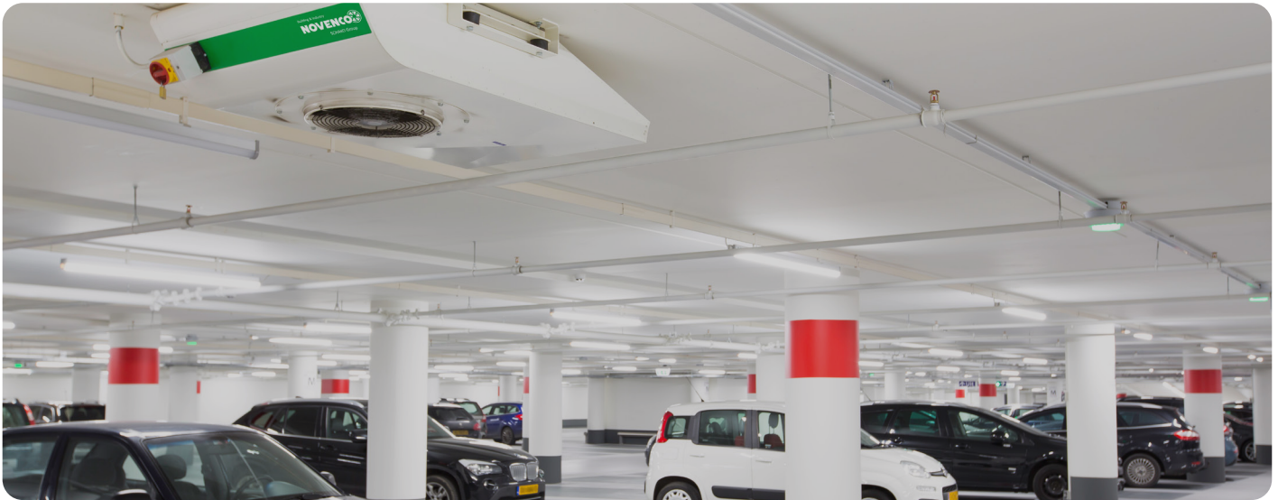
Air distribution across all five levels of the car park is handled by 42 CGF-500 centrifugal jet fans
