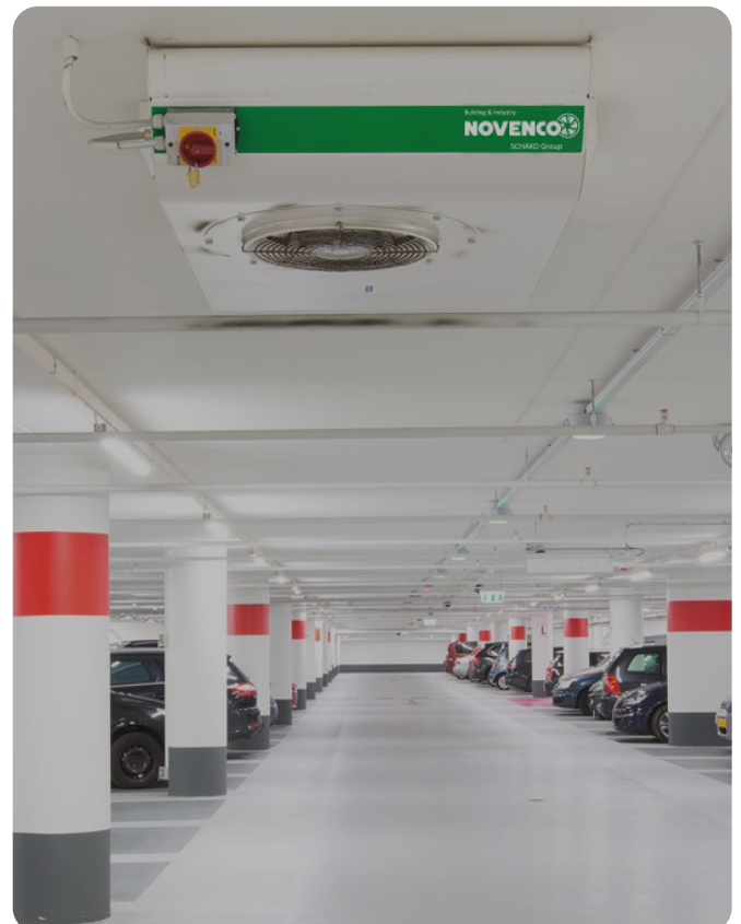
CGF-500 jet fan with under 27 cm installation for maximum car park clearance
