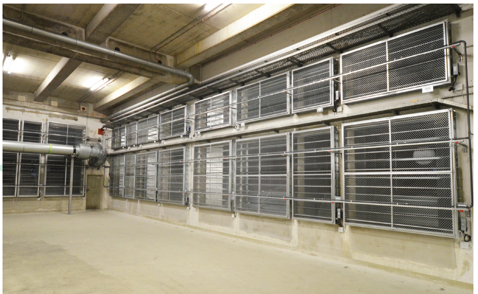
Blow-out chamber with louvre dampers Thanks to the ducts, the flow velocity is kept up to the dampers meaning no more energy is wasted
