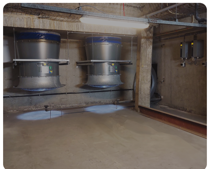
Post-installation: Compact, energy-efficient ZerAx fans
