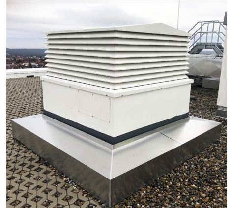
Rooftop louvre hood with high-speed actuator, designed for 0.7-second response, ensuring immediate airflow regulation and system stability
