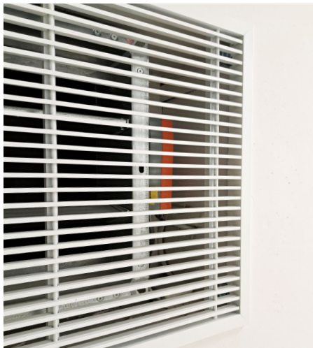
Corridor-mounted combination damper and outlet grille, delivering precise airflow and homogeneous pressure as part of the system
