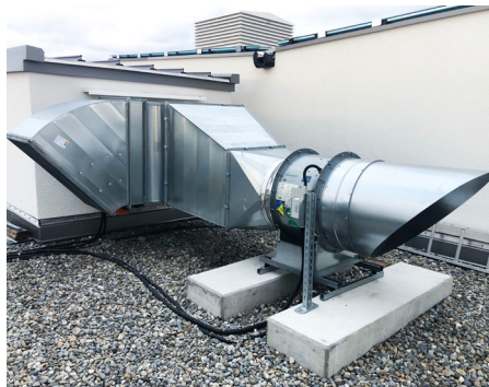
New bypass-solution with NOVENCO NovAx fan installed stalled on the rooftop for optimal airflow and performance
