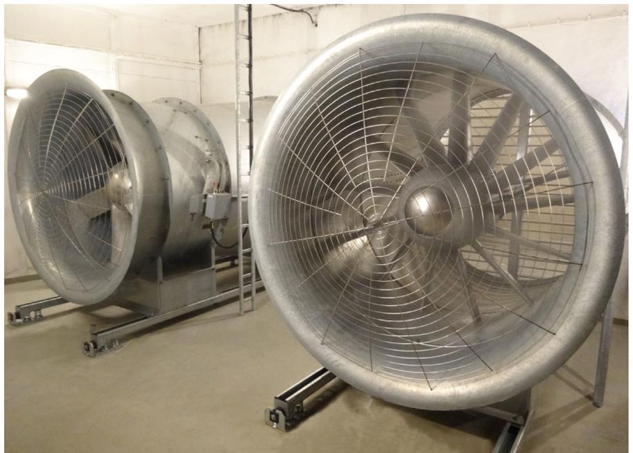
New high efficiency ZerAx® axial flow fans installed at Sima Power Station
