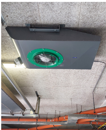
NOVENCO jet fans installed directly on the ceiling for maximum efficiency and space savings
