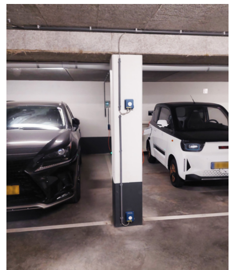
CO/LPG detection system ensures continuous monitoring and safety
