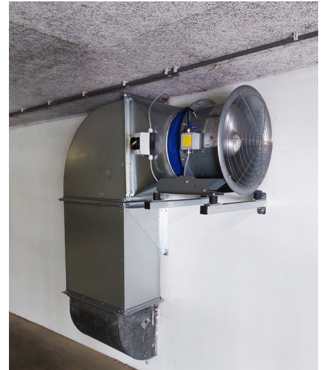
After: modern jet fan solution – reliable and energy-efficient
