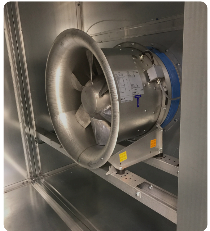
ZerAx® axial flow fan in AHU section
