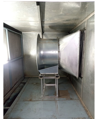
NOVENCO ZerAx axial fan as of 2024 – here the supplied energy is much more optimally utilised, since the static pressure is kept, and the total pressure is increased due to the high dynamic pressure. The space-performance ratio is relatively small, and the air volume is high.
