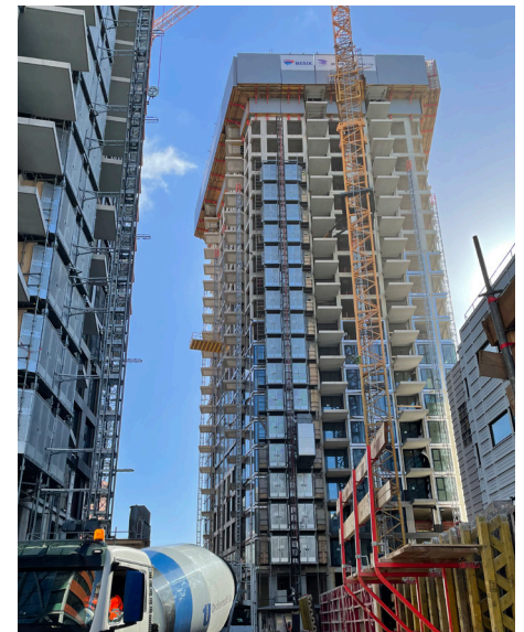
Completion of the project is expected in 2022
