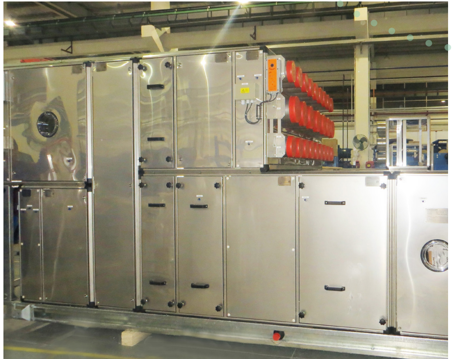
Air handling unit with NOVENCO® ZerAx® fan inside
