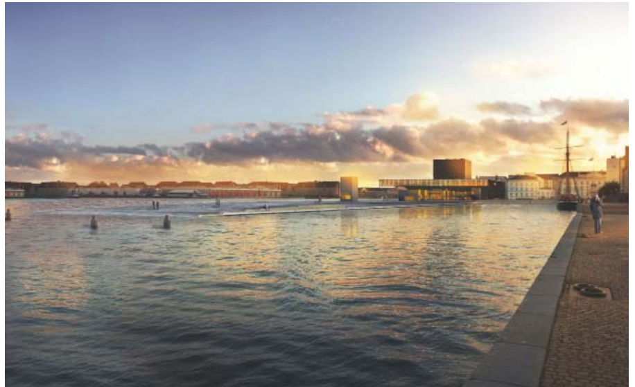
The Kvaesthus car park is a very unique construction with its 3 levels built below water surface
